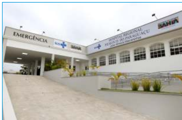
Hospital Regional Piemonte do Paraguaçu - Itaberaba/Ba
